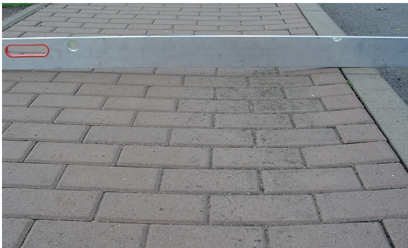
Fig.: Depressions in the surface, formation of ruts
